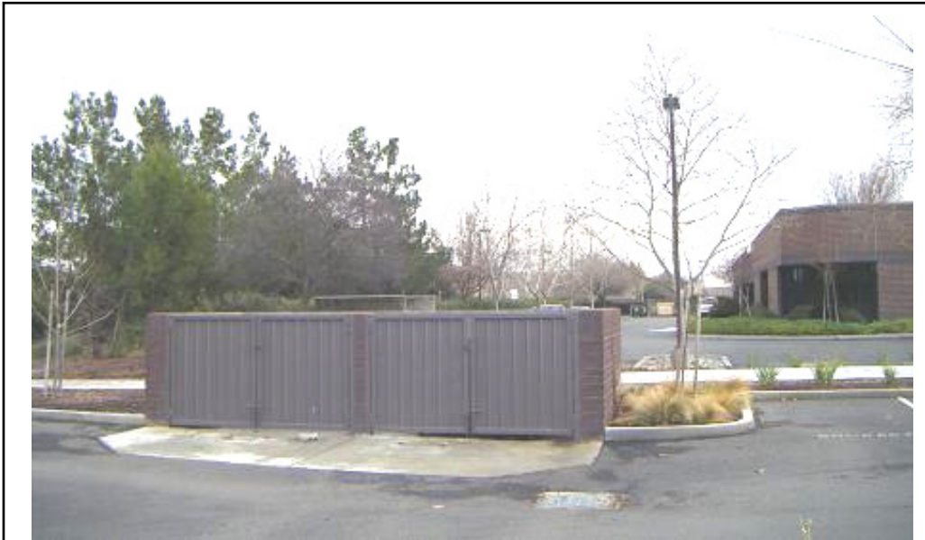
Figure 23: This trash collection and recycling enclosure uses similar building materials and colors to blend in with the primary buildings.
