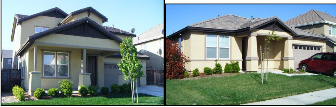
Both homes have a porch as the prominent feature. A recessed second story (left) makes homes of varying sizes architecturally compatible.
