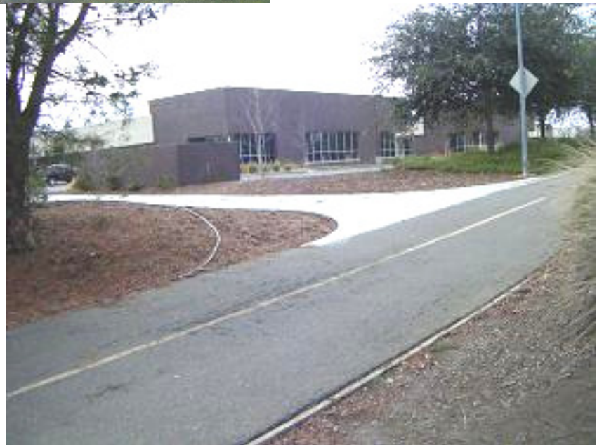
Figure 10: The same complex of buildings has a walking and bicycle path that connects to a grocery store, restaurants and a park.
