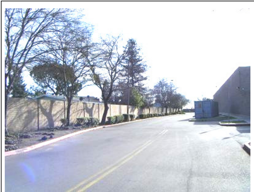
Figure 7: A masonry wall and a row of trees buffer the residential neighborhood from the industrial use. The loading docks and storage area are located away from the residential use.
