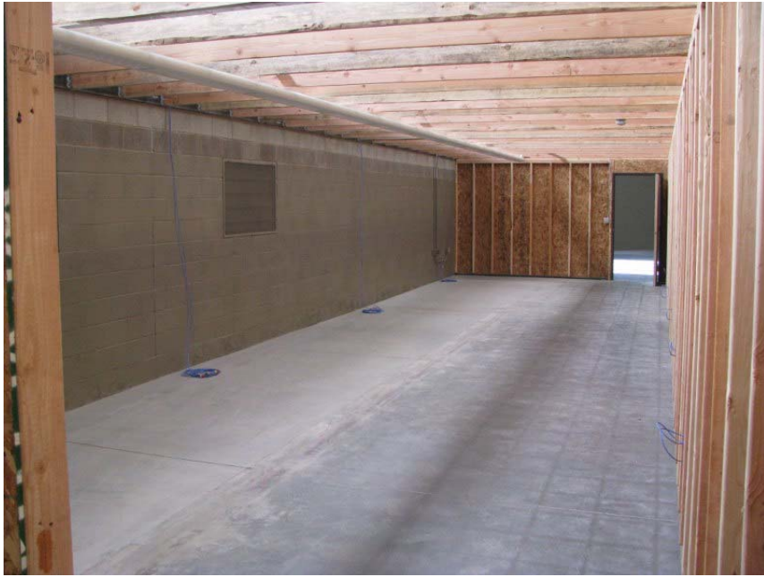
2nd Street temporary library, early construction, staff office area part 1
