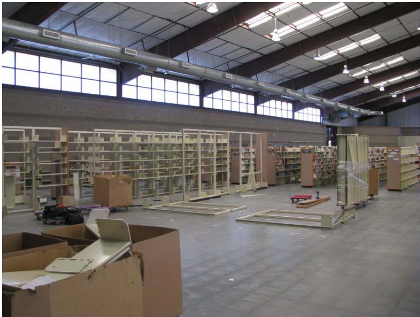
2nd Street temporary library book stacks being installed part 1
