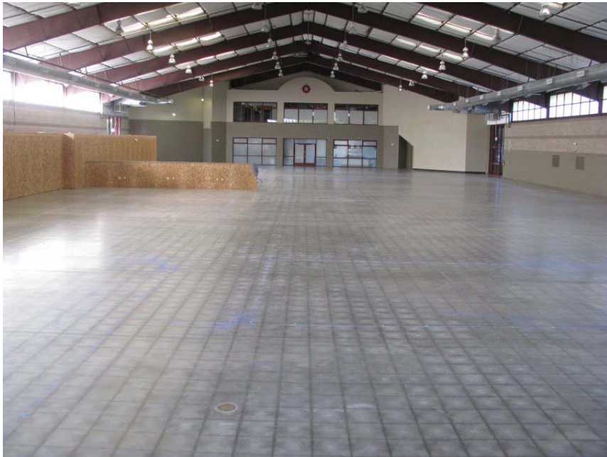
2nd Street temp library Early construction 1
