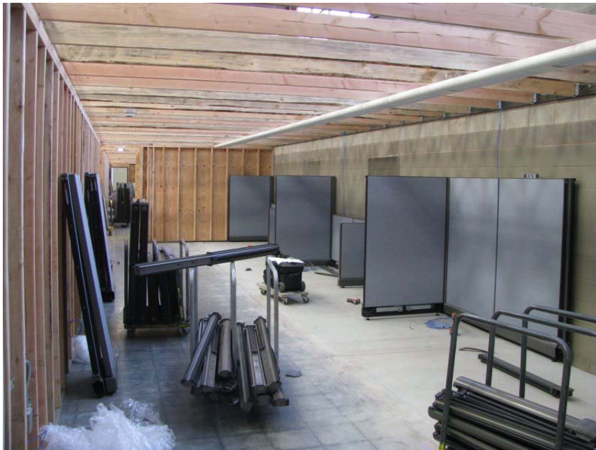
2nd Street temporary library, early construction, staff office area part 2
