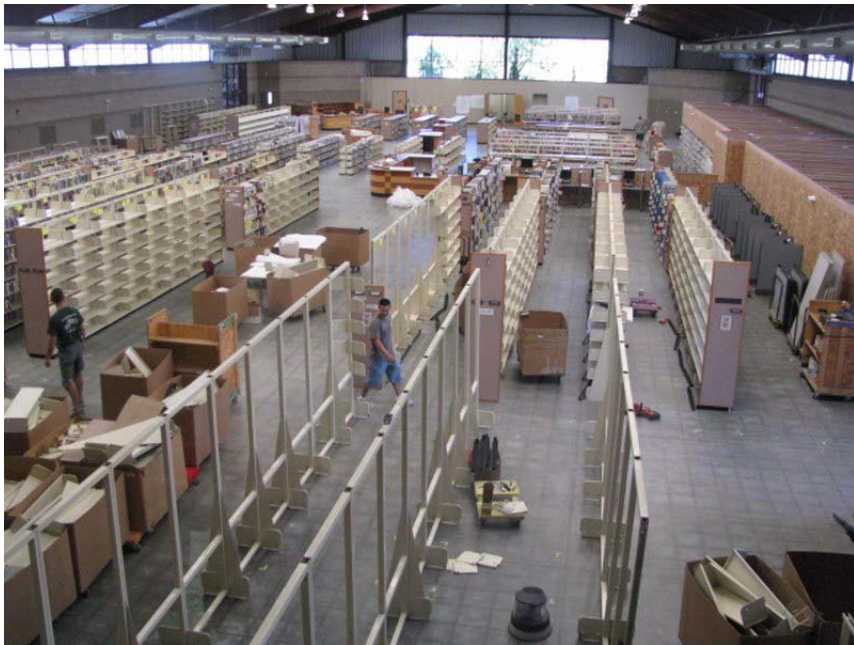
2nd Street temporary library book stacks being installed part 2
