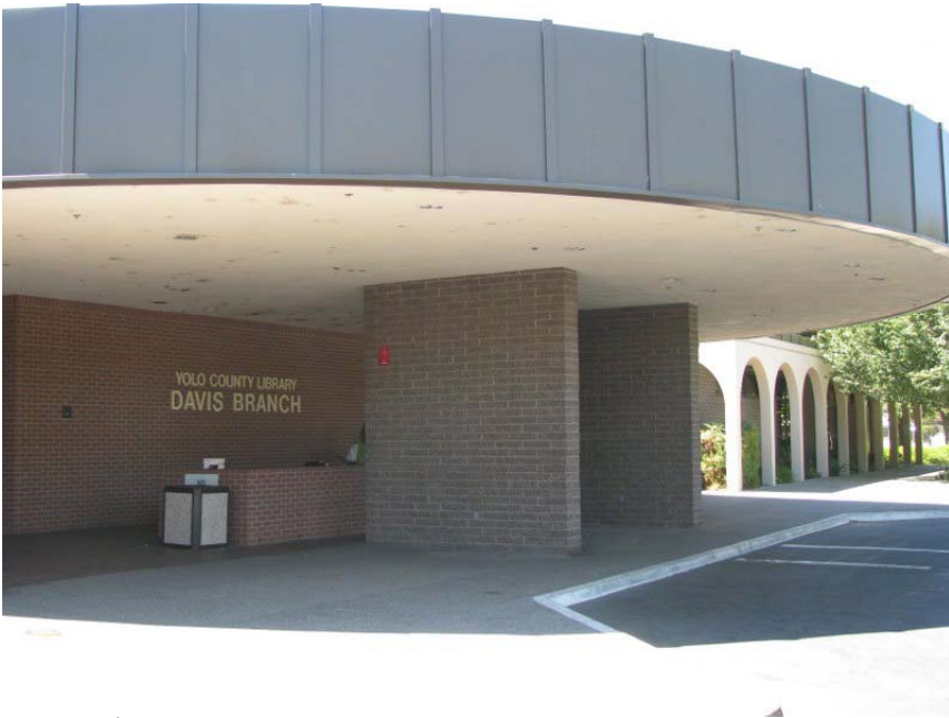
East 14 th Street - East side before renovation.
