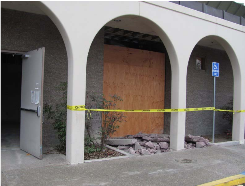
East 14 th Street - Early renovation - Staff and Friends entrances.
