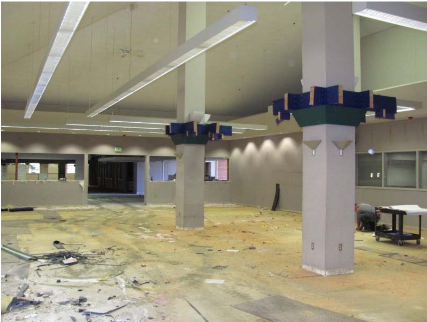
East 14 th Street - early demolition, Children's room.
