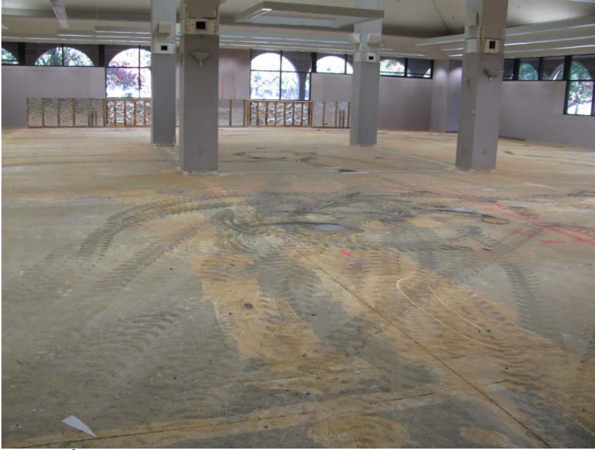
East 14 th Street - early demolition, Adult non-fiction and reference areas.
