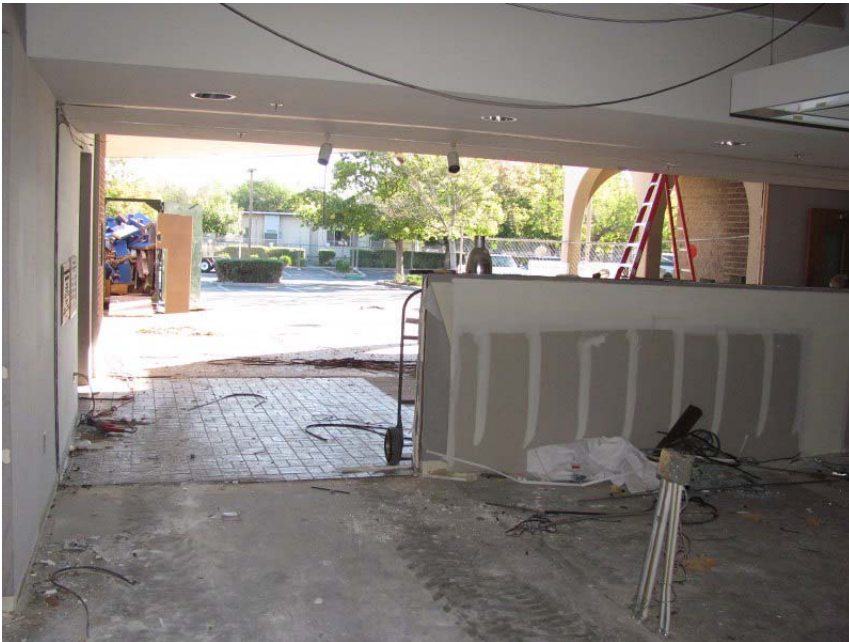
East 14 th Street - Early Construction, Main Entrance Interior looking out.
