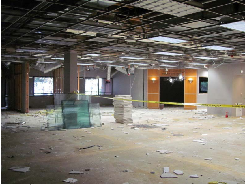
East 14 th Street - early demolition, looking toward the Hughes room.
