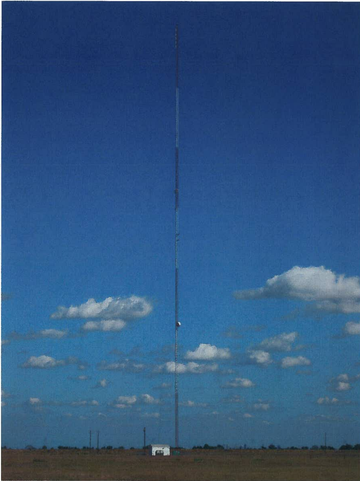
Existing 500-foot radio tower located off County Road 102, just south of the Mountain Valley Golf Center (APN: 042-010-68, approved in 1992)
