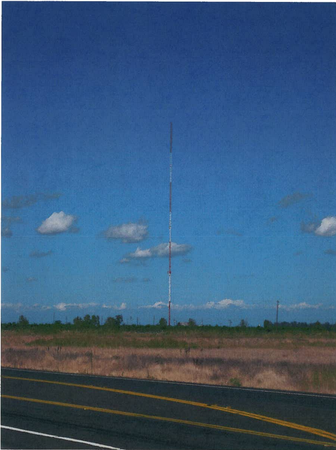
Existing 538-foot radio tower located off County Road 102 and County Road 29 (APN: 042-120-03, approved in 1992)
