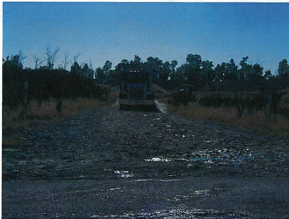
Semi-Truck exiting the project site through the ingress/egress point on the east side of County Road 100B
