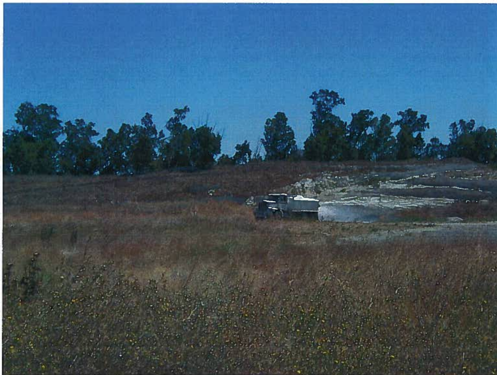
Water truck providing water to the project site access road
