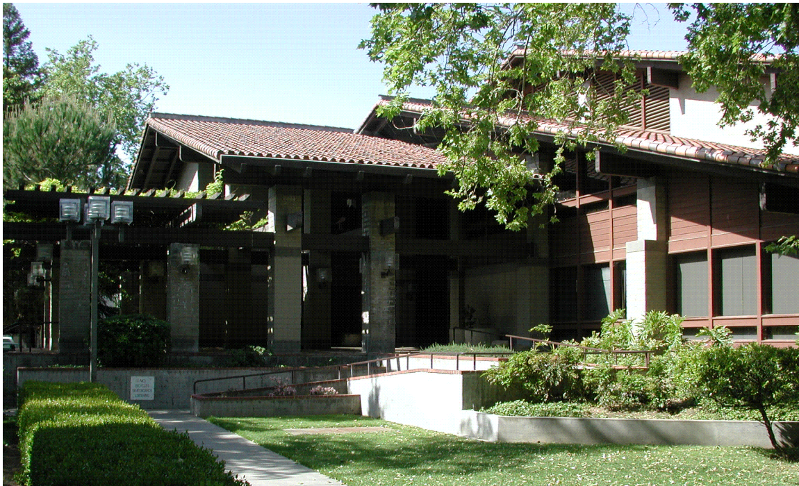
Erwin Meier Administration Building
