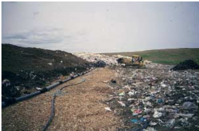
Image 3-1: Horizontal LFG and leachate injection lines installed and being covered by shredded tires.
