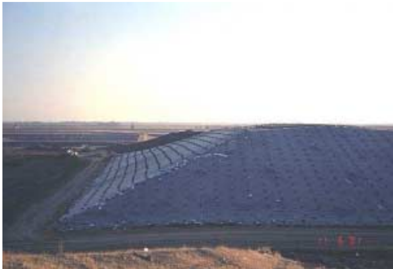
Image 3-3: Northeast anaerobic surface liner
