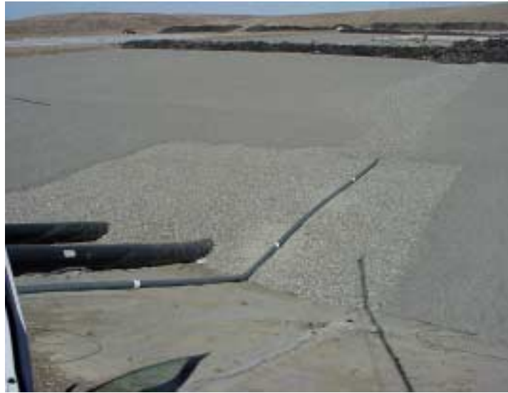
Image 5: Gravel drainage layer and leachate collection sump
