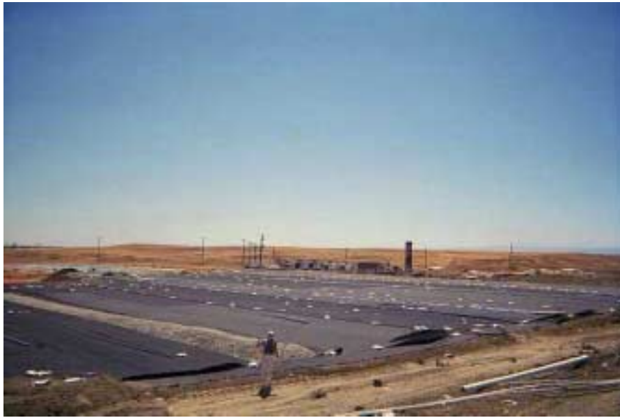
Image 8: Aerobic liner ready for shredded tire operations layer and waste placement
