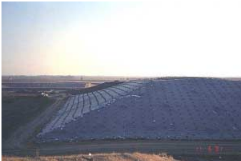
Image 3: Northeast anaerobic surface liner
