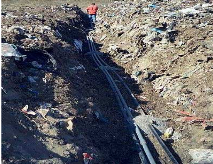
Image 9: Leachate injection laterals in trench
