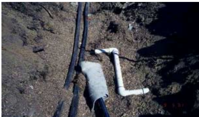
Image 11: Moisture, temperature, and tube installation
