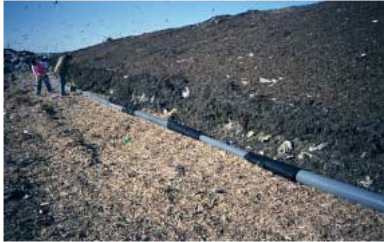
Image 2: Horizontal LFG collection line installation
