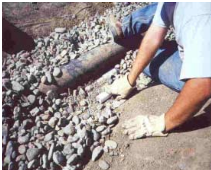
Image 15: Pressure tubes installed in LCRS trench
