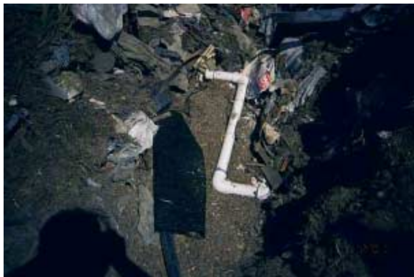
Image 4: Moisture, temperature, and tube installation
