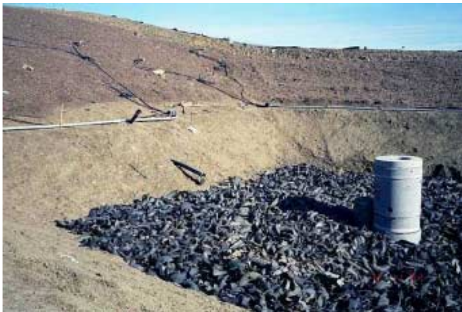
Image 12: Aerobic sump installed and ready for backfill
