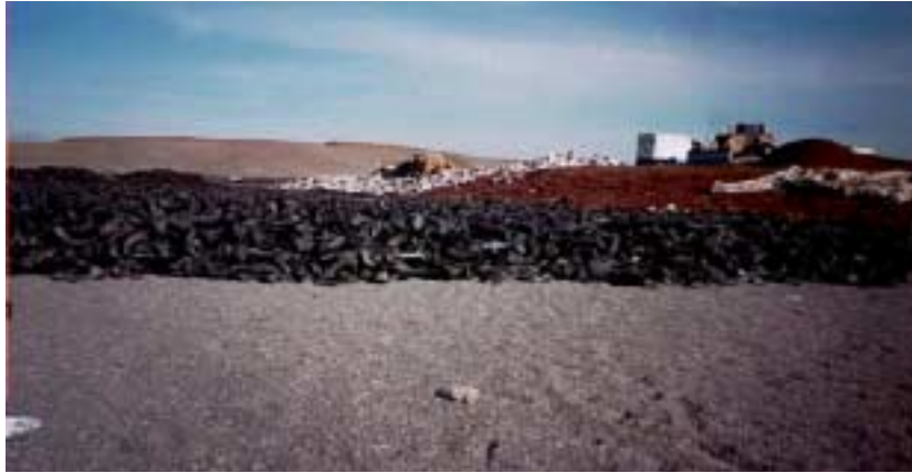
Image 14: Shredded tire operations layer
