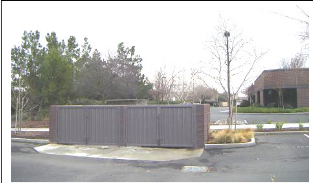
Figure 23: This trash collection and recycling enclosure uses similar building materials and colors to blend in with the primary buildings.
