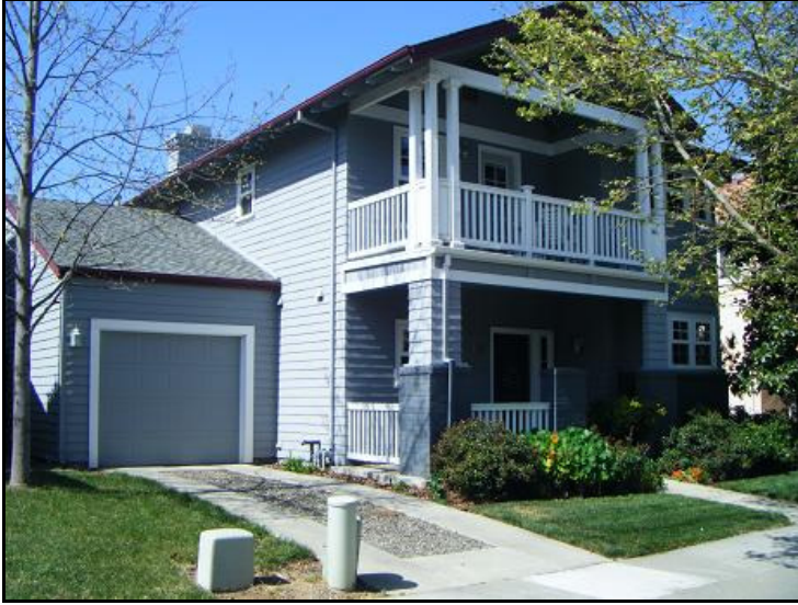
The driveway for this house is semi-pervious, using gravel in the center, to avoid excess runoff. The garage is recessed from the house, making the front porch and entry the prominent view.
