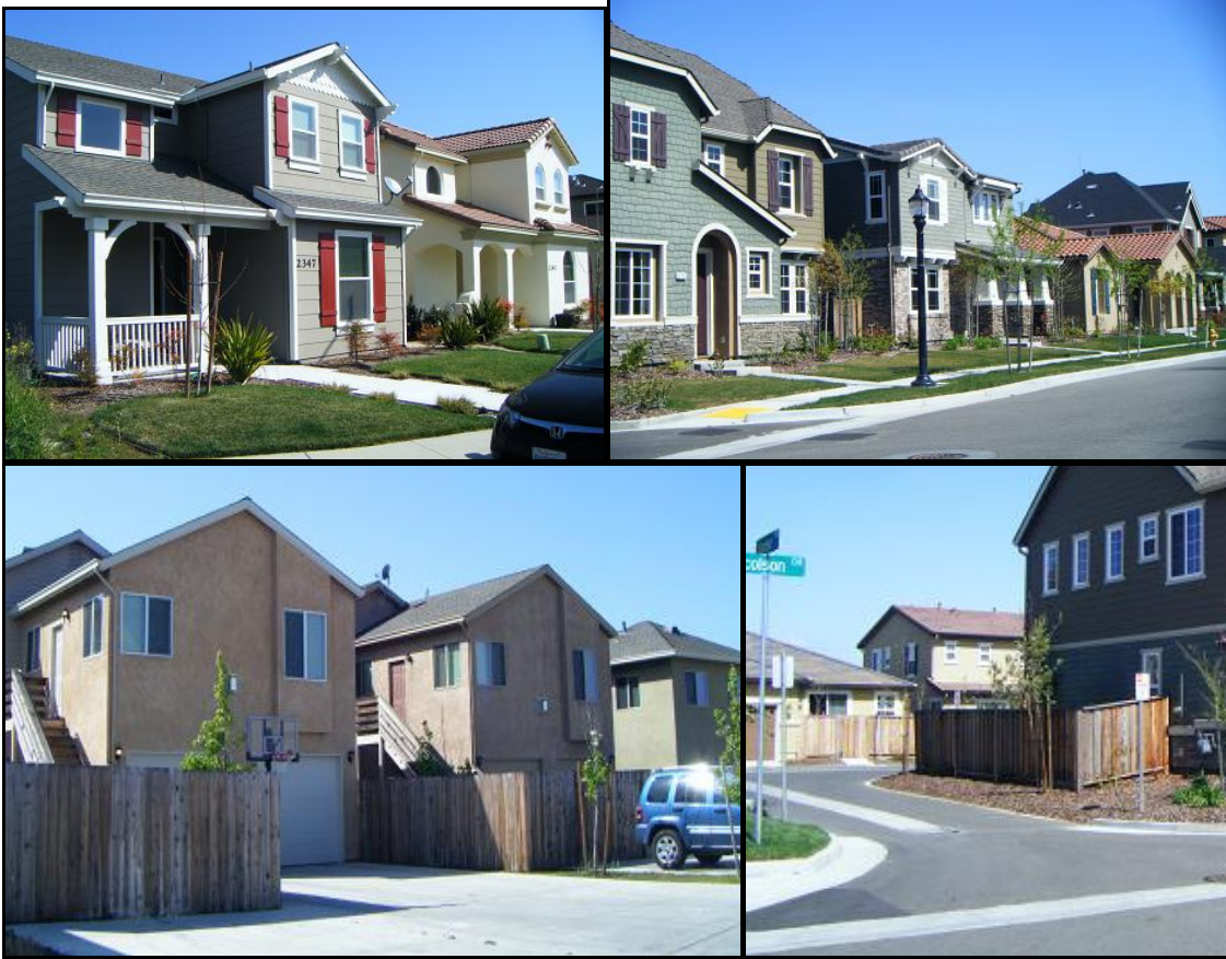
Compact development can make use of garages located on a private alley to the rear of the homes. The lack of garages visible to the street makes for a more inviting human scaled neighborhood (above right and left). Windows overlooking the alley increase safety (lower left). One private alley serves garages for homes on two different streets (lower right).
