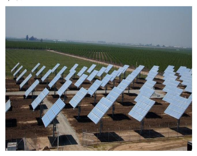
Alongside the sprawling grove of pistachio trees at Nichols Farms near Fresno, a 6-acre solar-panel installation is now up and running. The 1-megawatt concentrating photovoltaic project is connected to the Southern California Edison grid and will produce enough electricity to cover 70% of the 50-year-old pistachio farm's demand.
