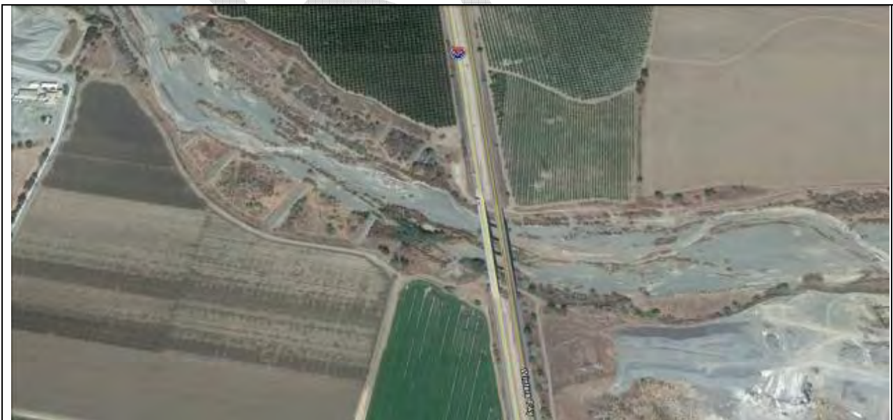
Figure 33 Interstate 505 Bridge (River Mile 21.0)
