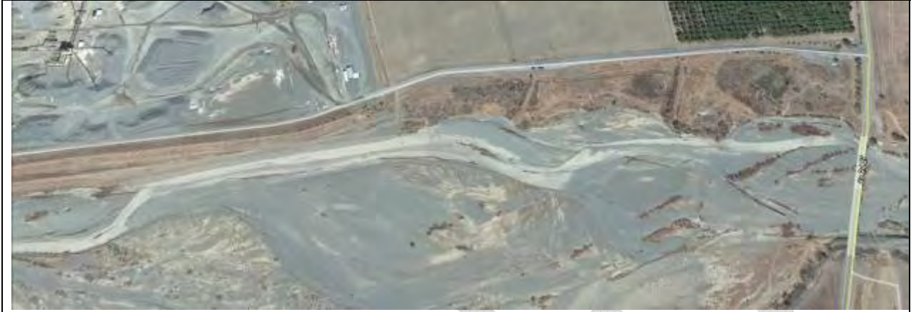
Figure 32 Esparto Bridge (County Road 87) River Mile 24.4
