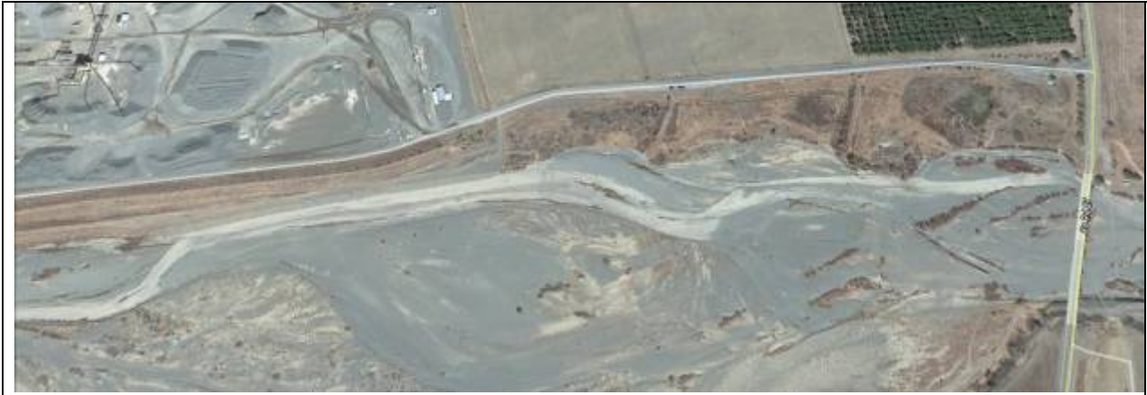
Figure 32 Esparto Bridge (County Road 87) River Mile 24.4
