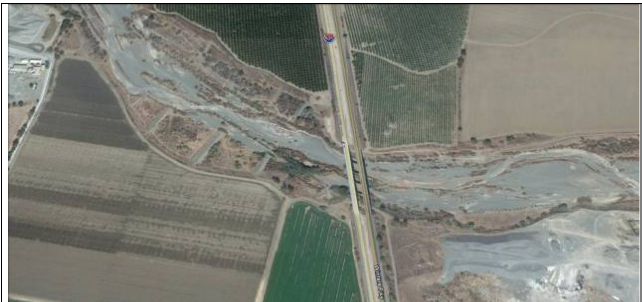
Figure 33 Interstate 505 Bridge (River Mile 21.0)
