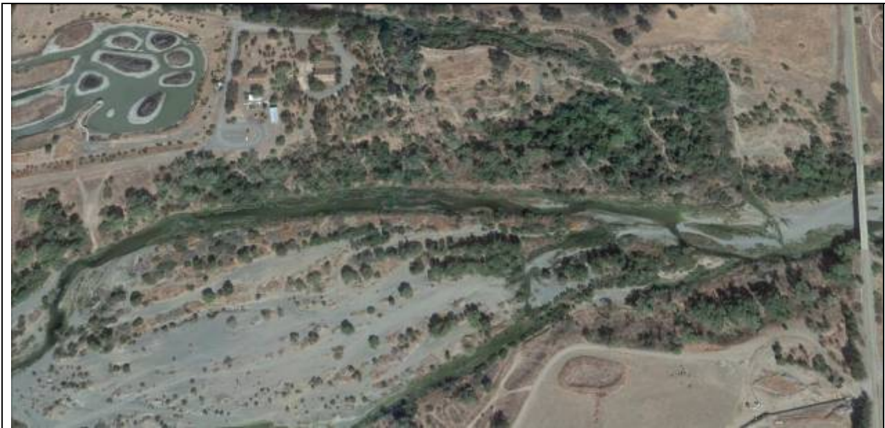
Figure 34 County Road 94b Bridge
