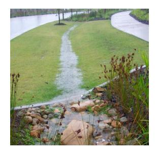
LID principles and practices, water can be managed in a way that reduces the impact of built areas and promotes the natural movement of water within an ecosystem or watershed. Applied on a broad scale, LID can maintain or restore a watershed's hydrologic and ecological functions. The County will review its Development Standards to incorporate LID standards as appropriate.
