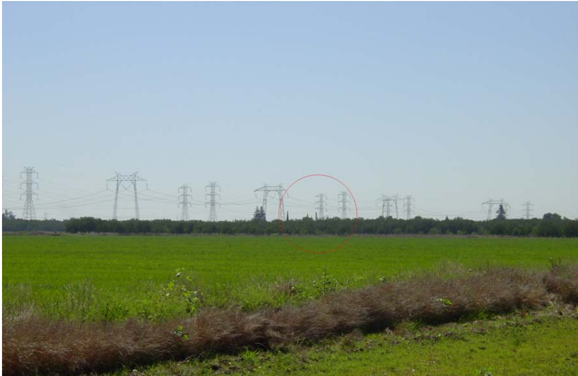
Tower 2 View D
