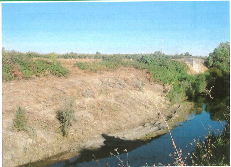
Dewey's by I-5 after cutting with excavator.
