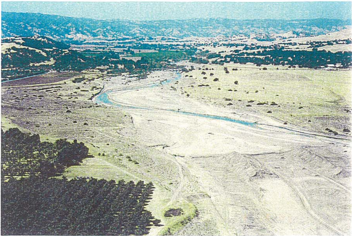
Looking Upstream Towards Capay Bridge (September 10, 1995)
