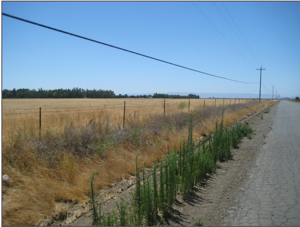
Photograph 1: View facing project site to the west, along County Road 35.
