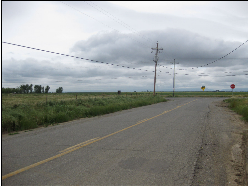
Photograph 5: View of transformer located at the northwest corner of project site, located at the intersection of County Road 104 and 35.
