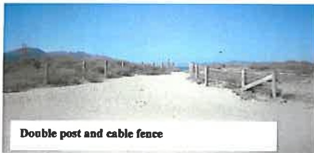
Double fence: post and cable with field fencing & buffer
