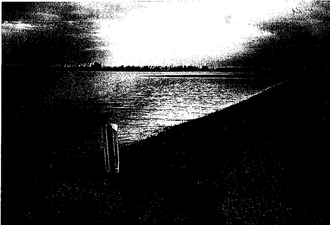
FIGURE 3-22- STORMWATER BACKUP (VIEW TO WEST FROM AVIATION AVENUE)
