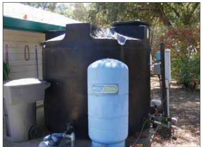
PHOTO 16: 2,500-gallon water holding tank and water softener located behind the garage.
