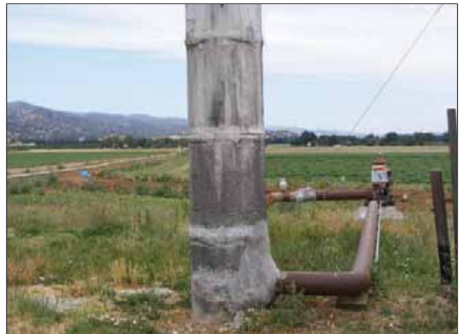
PHOTO 12: One of two agricultural wells located on the Subject Property.
