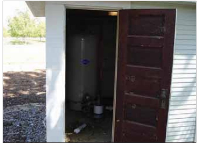
Door to utility room located on Parcel 6
