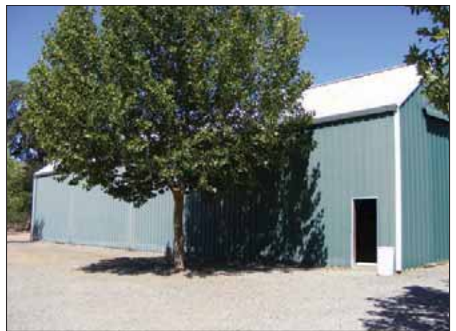
POTO 10: Metal shop building
