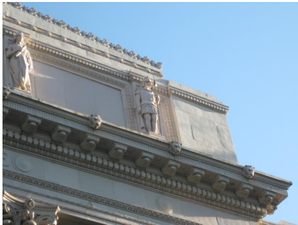
Image 15 – South Façade Detail
