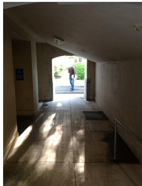
Image 8 – Main Basement Entry Below Grand Entry Stairway
