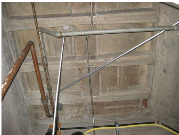
Image 75 – Un-braced Utilities
