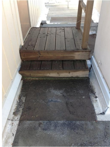
Image 34 – Wood Stair at Roof
