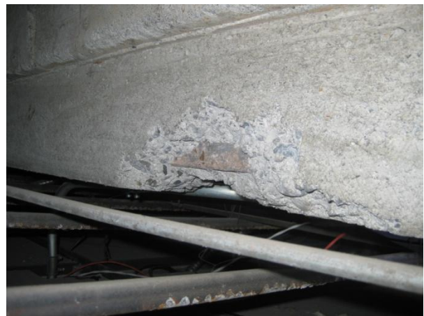
Image 72 – Exposed Rebar
