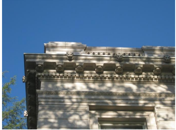
Image 18 – South Façade Detail
