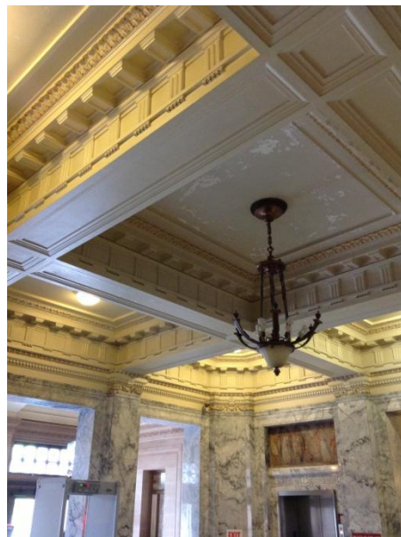
Image 56 – First Floor Rotunda Ceiling
