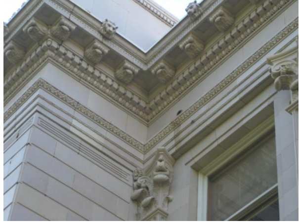
Image 14 – South Façade Detail
