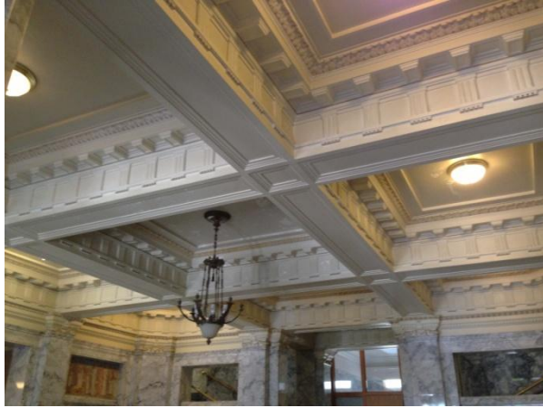
Image 57 – First Floor Rotunda Ceiling
