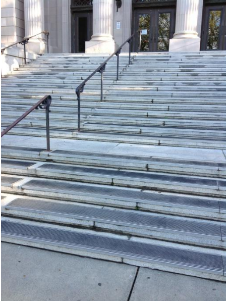
Image 5 – Grand Entry Stairway
