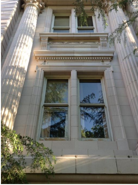
Image 13 – South Façade Detail
