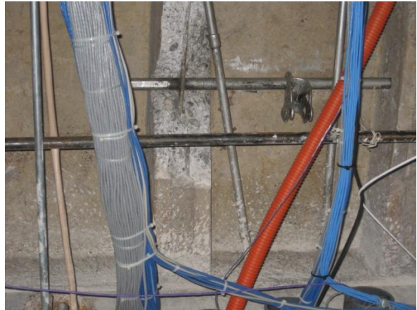
Image 74 – Exposed Rebar
