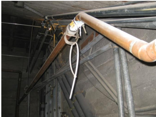
Image 79 – Un-braced Utilities
