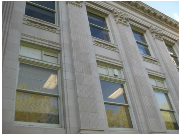
Image 16 – South Façade Detail
