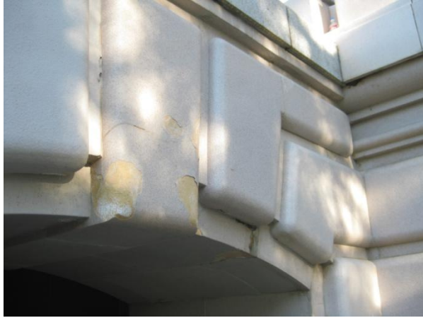
Image 17 – South Façade Detail
