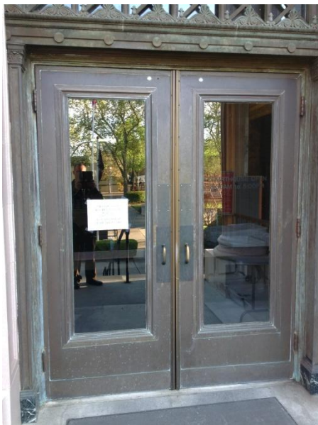
Image 7 – One of Three Main Entry Doors
