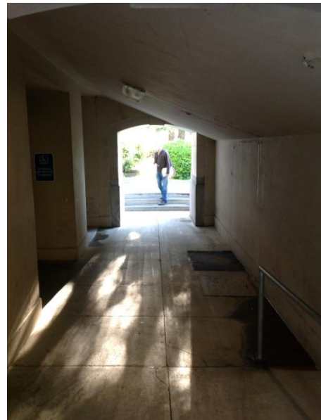
Image 8 – Main Basement Entry Below Grand Entry Stairway
