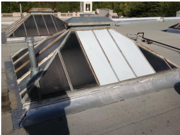
Image 39 – Skylight Over Rotunda
