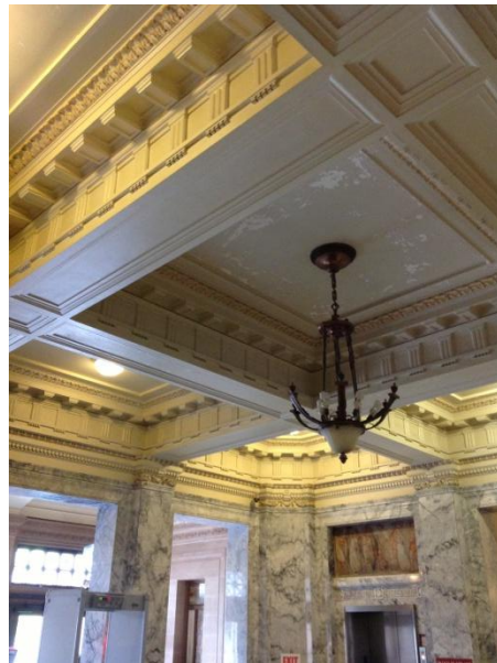
Image 56 – First Floor Rotunda Ceiling
