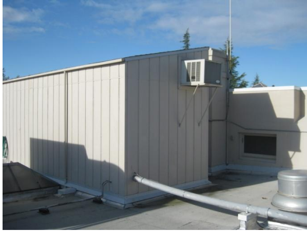
Image 37 – IT Room at Roof
