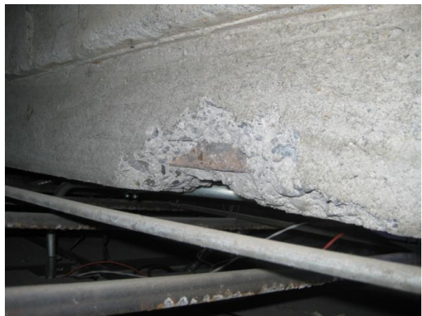
Image 72 – Exposed Rebar
