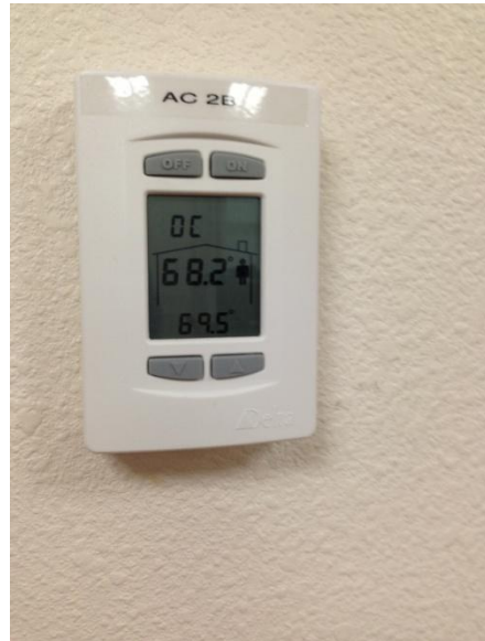
Image 76 – Delta Control Thermostat
