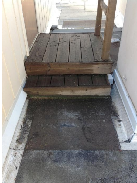
Image 34 – Wood Stair at Roof
