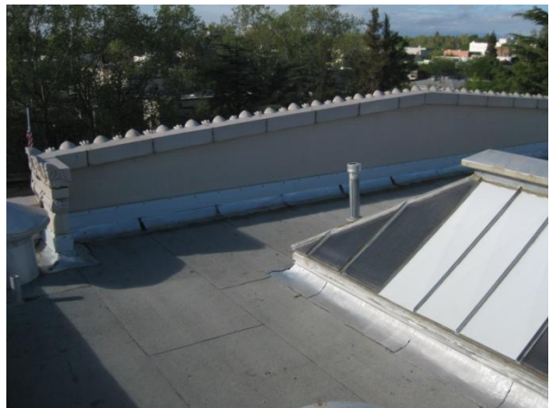
Image 40 – Skylight Over Rotunda
