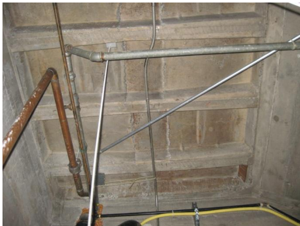
Image 75 – Un-braced Utilities
