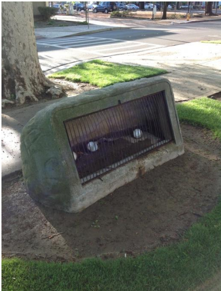
Image 3 – Faux Rock Lighting Enclosure
