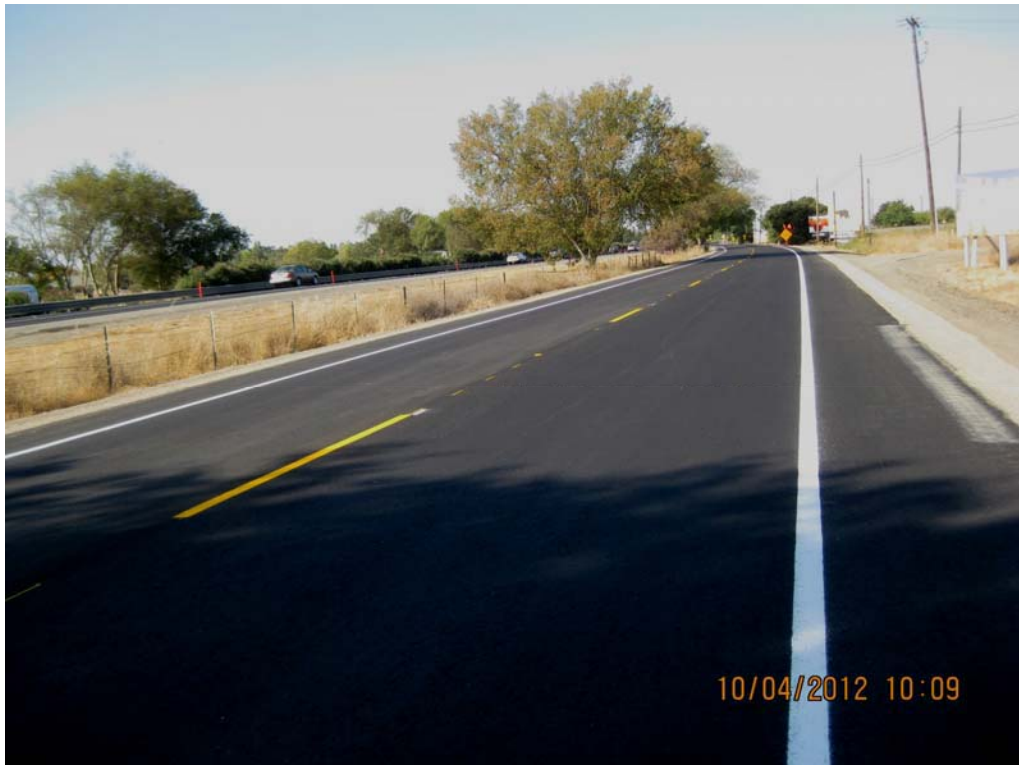
Post construction photo
