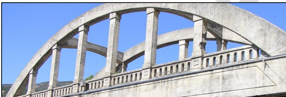
Vertical Hanger Elevation View (Span 1 right side)
