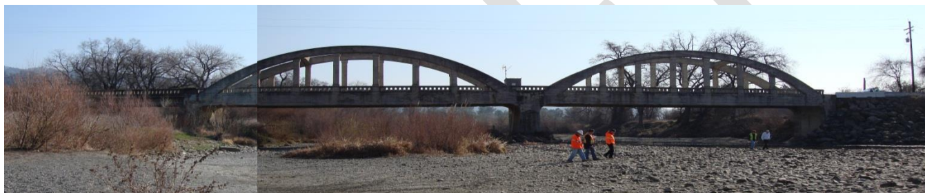
Elevation View of the Existing Bridge
