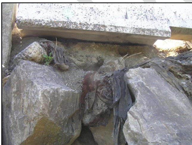
K-Rail placed on top of Abutment 1 RSP backfill
