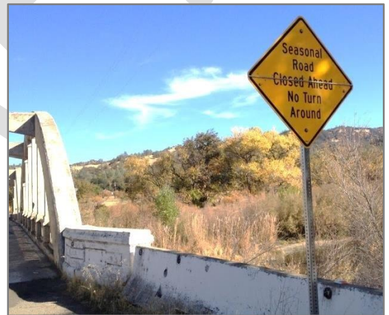
Seasonal Road Closed Sign
