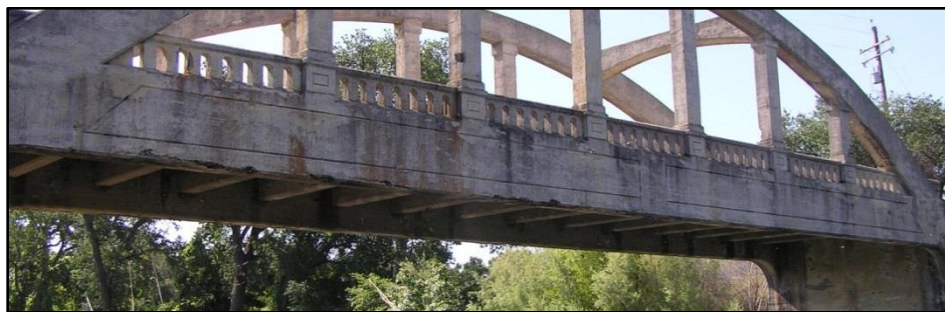
Span 1 elevation view – Tie Girder at span 1 left side
