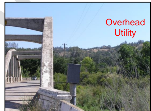
Overhead Utility on Eastside of existing bridge
