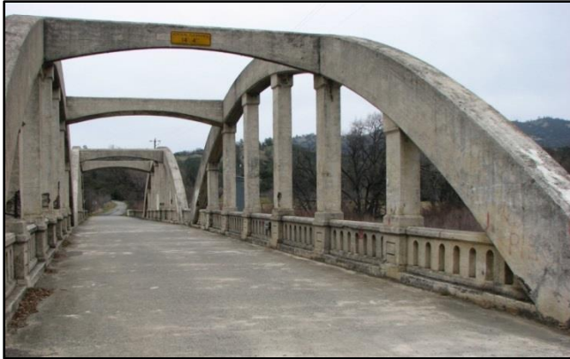
Original main Arch spans
