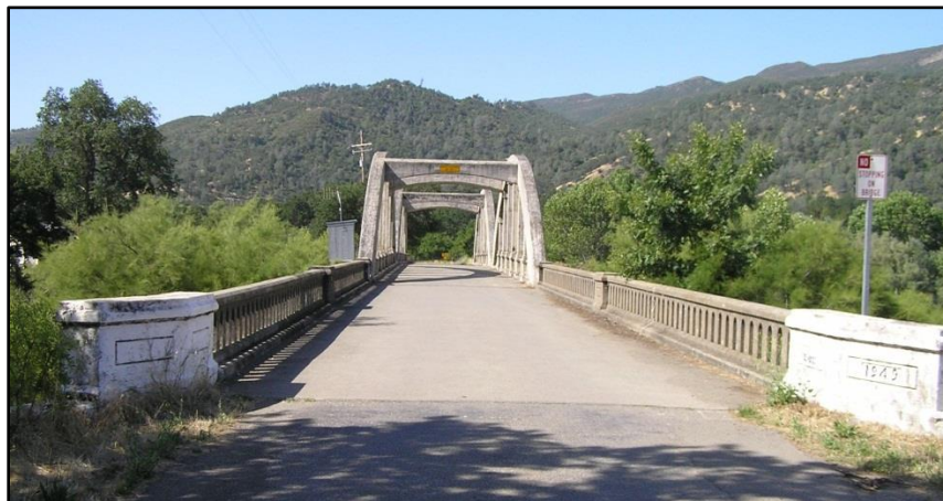
Rumsey Bridge viewed south-west from Abutment 5
