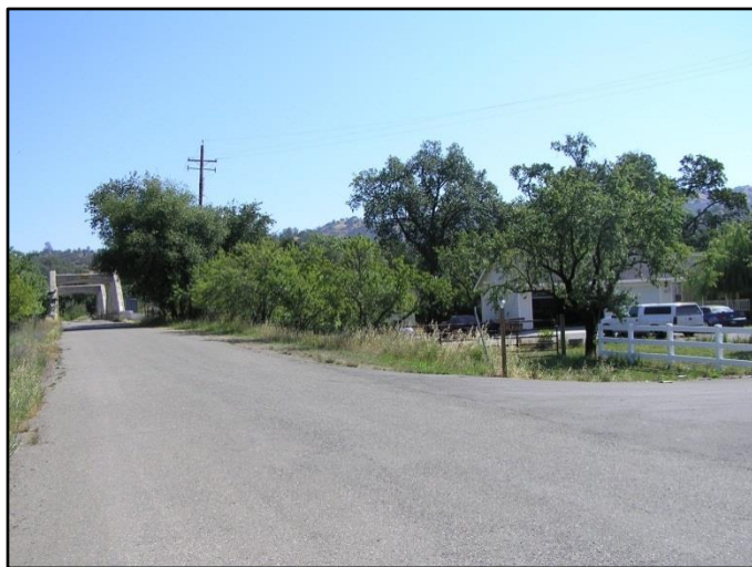
Southside Approach Roadway (before Beginning of Bridge)
