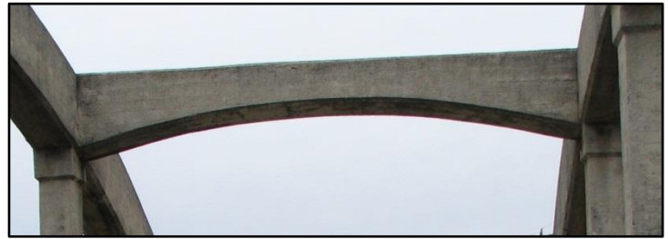
Portal Bracing (Span 1, 2 nd portal)
