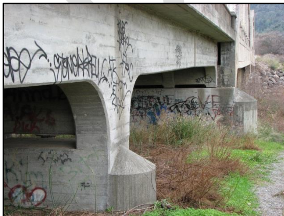
Pier 3 and Pier 4 (left side of bridge)
