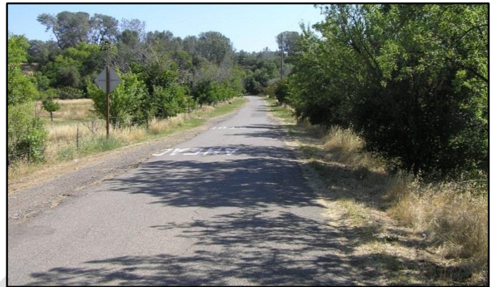
Northside Approach Roadway (from End of Bridge)
