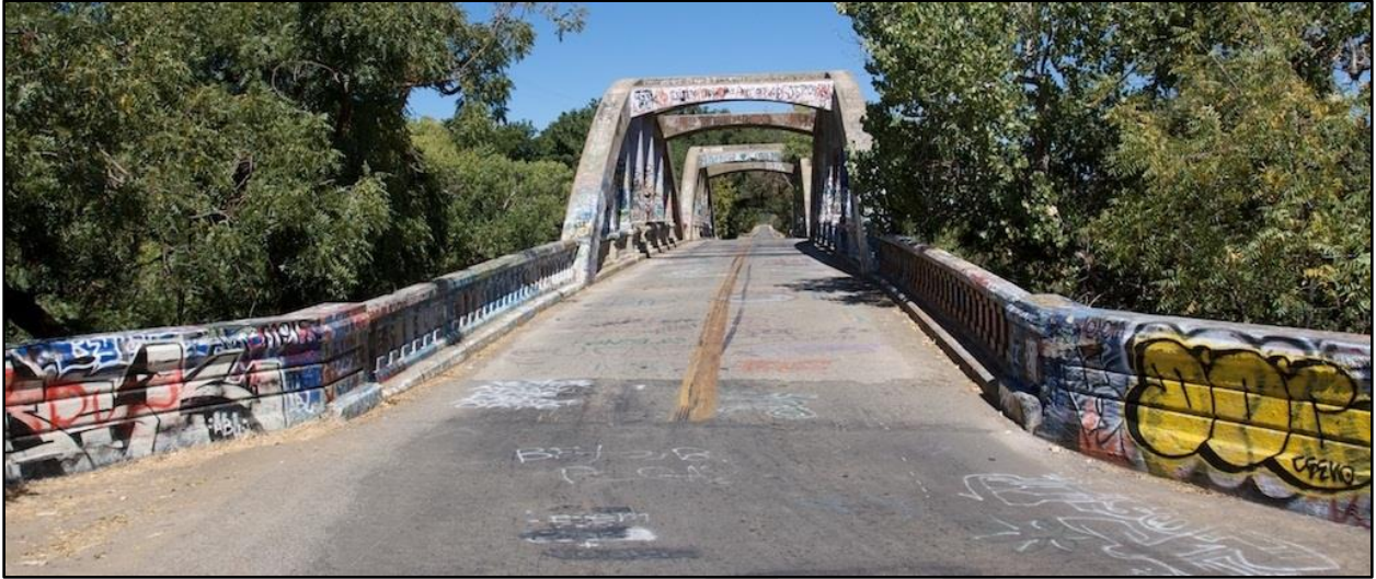
Stevenson Bridge, standing at Abutment 1, looking north
