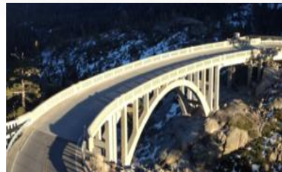
Donner Summit Bridge Nevada County, CA
