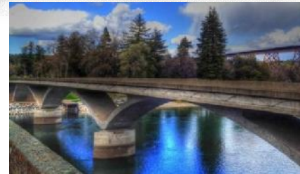
Diesloehorst Bridge Redding, CA
