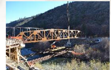
Klamath River Bridge
