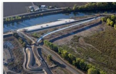
Tisdale Bypass Bridge Sutter County, CA
