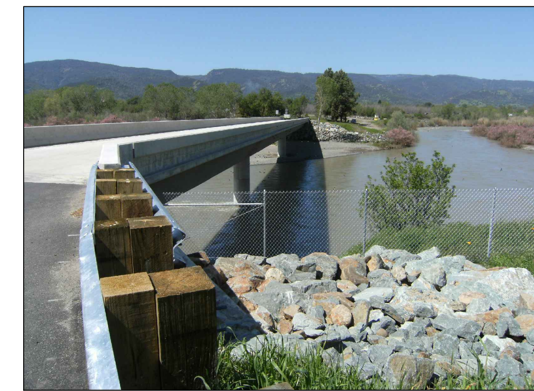
GUINDA BRIDGE (SIMILAR)
