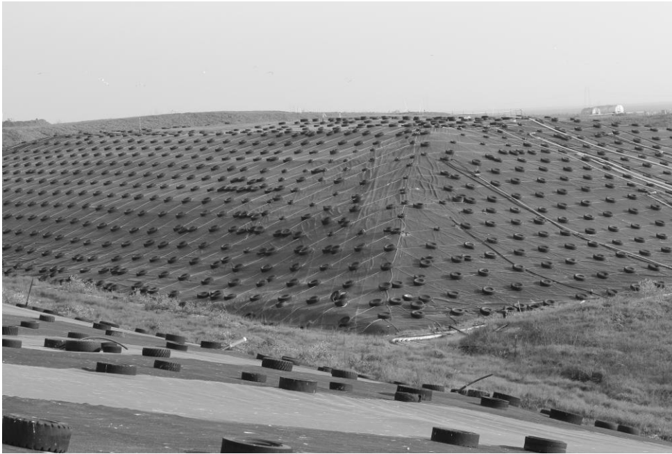
Figure 1: Yolo County Central Landfill anaerobic bioreactors showing use of tires to secure vinyl covering.
