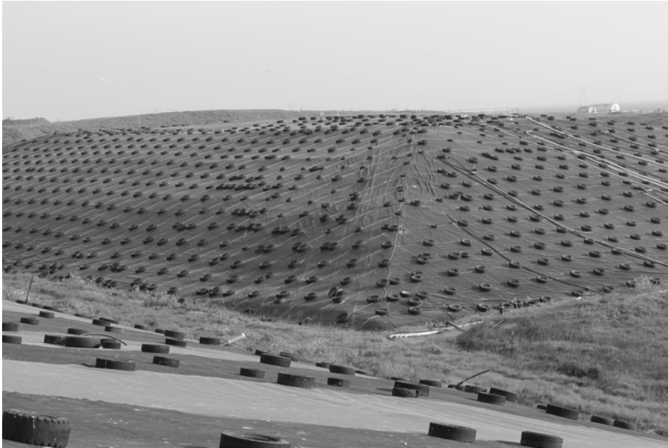
Figure 1: Yolo County Central Landfill anaerobic bioreactors showing use of tires to secure vinyl covering.
