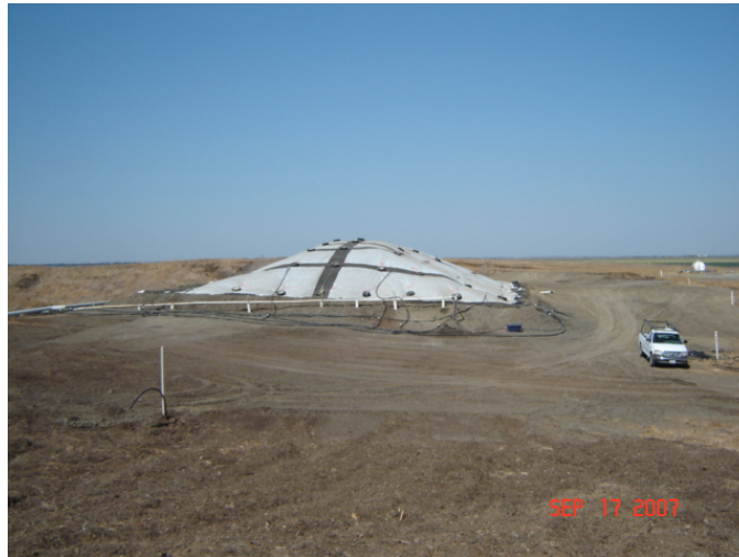
Picture 9: Completed surface liner system
