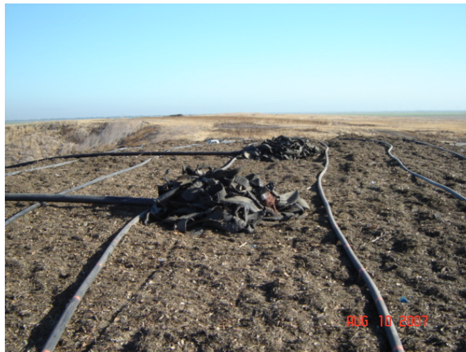
Picture 8: Horizontal air injection wells on layer 1 and 5.
