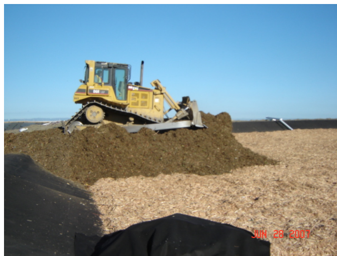
Picture 3: Placement and compaction of green waste with D6 bulldozer
