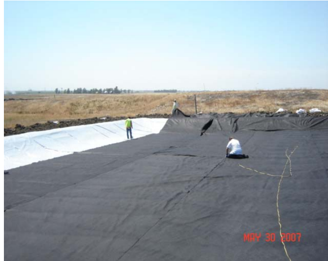
Picture 2: Installation of base liner and protective geotextile
