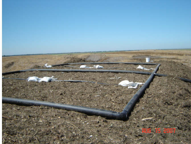
Picture 7: Gas collection lateral above layer 4 of waste
