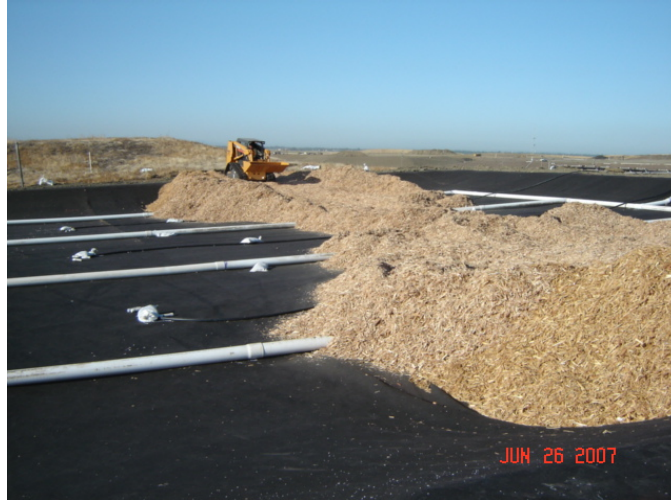
Picture 4: Placement of wood chips over the base liner
