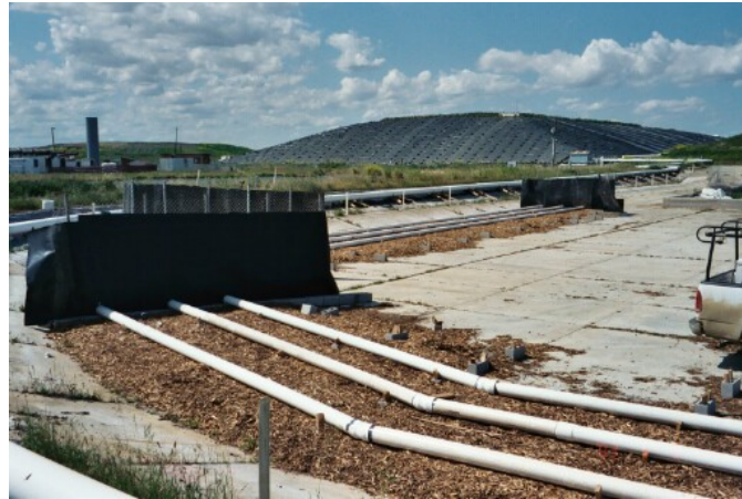
Picture 13: Biofilter #2 gas pipe installed prior to placement of biofilter material
