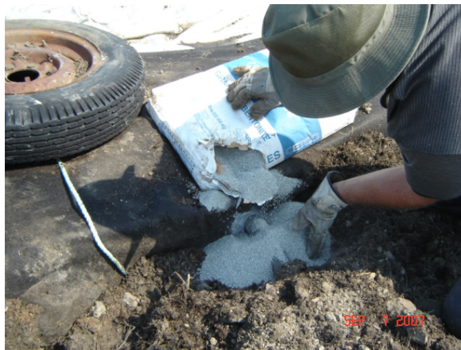
Picture 11: Bentonite placed around pipe penetrations to seal potential gas leaks
