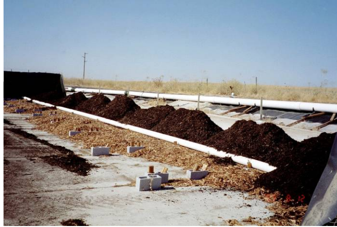
Picture 12: Biofilter #1 gas pipe installed prior to placement of biofilter material
