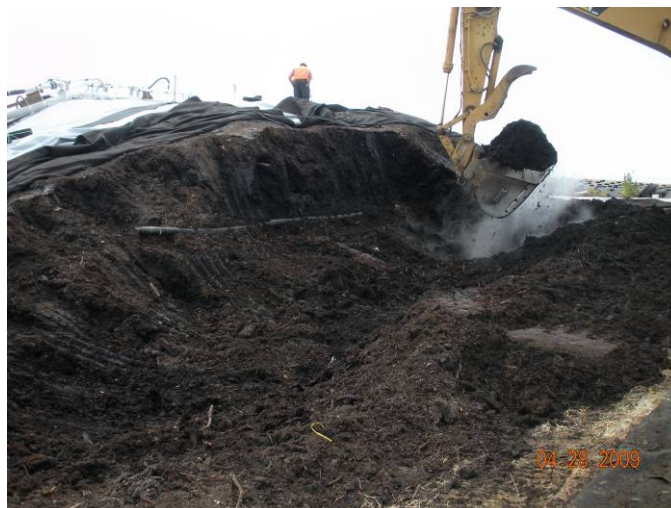
Picture 15: Excavation of digester cell
