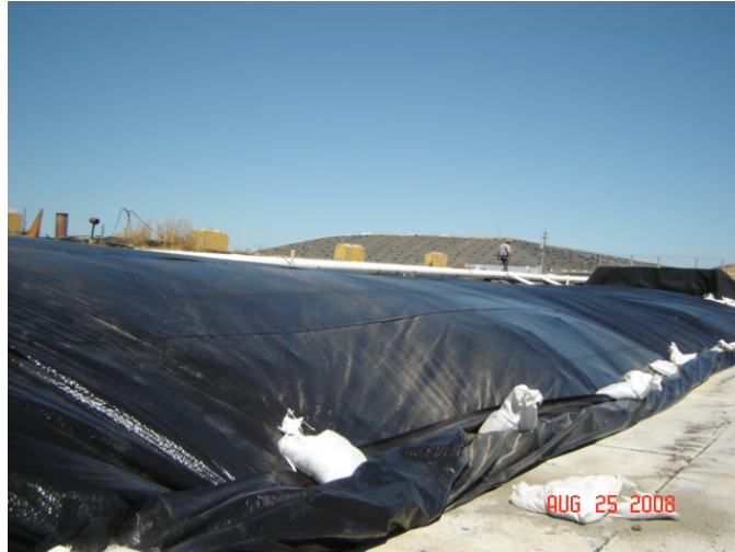
Picture 14: Biofilter cover liner installed and sealed around edges
