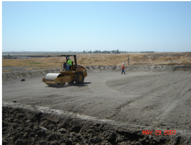
Picture 1: Compacted clay below the digester base liner
