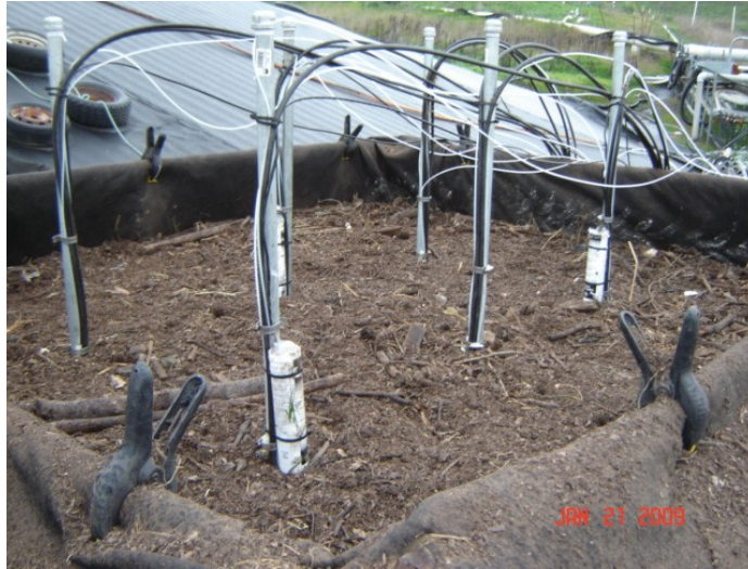
Figure 8. Nearing the end of addition of biocover material. Sensors shown for layer 2.
