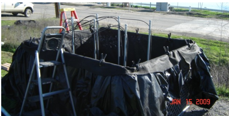
Figure 4. Biocover cell with metal rods inserted for support of sensors and tubing.
