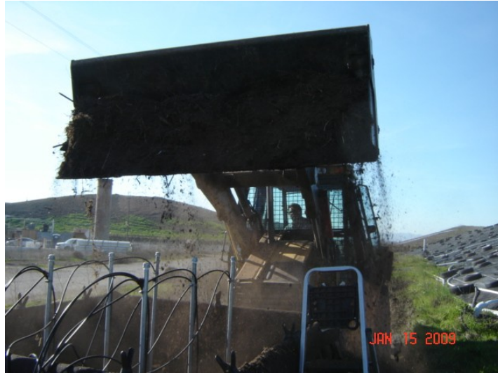
Figure 7. Filling biocover cell with aged and fresh green material.
