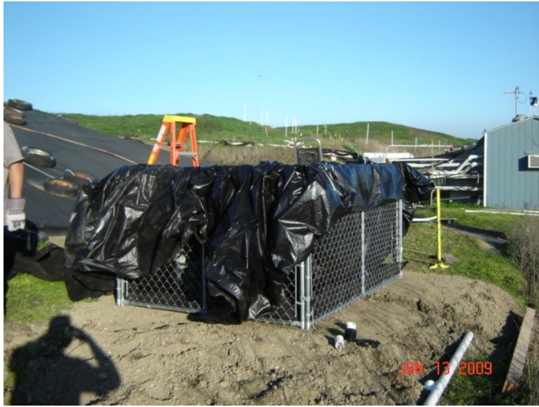
Figure 2. Chain link fencing used as structure for biocovers.
