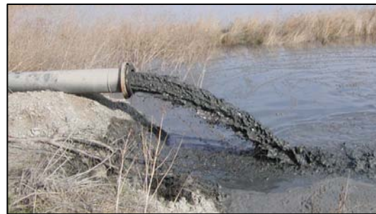
Example of Dredge Discharge
