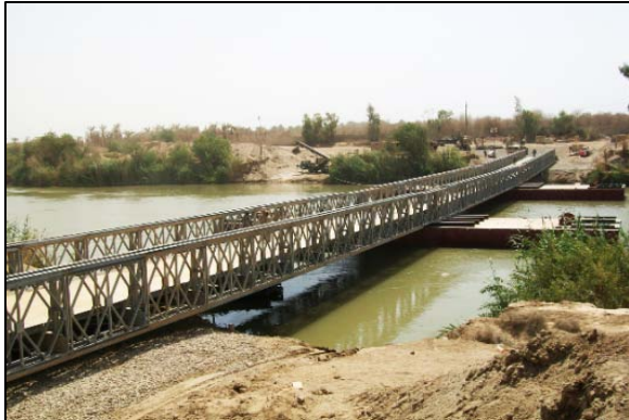
Typical Floating Bridge
