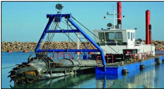
Example of Hydraulic Dredge
