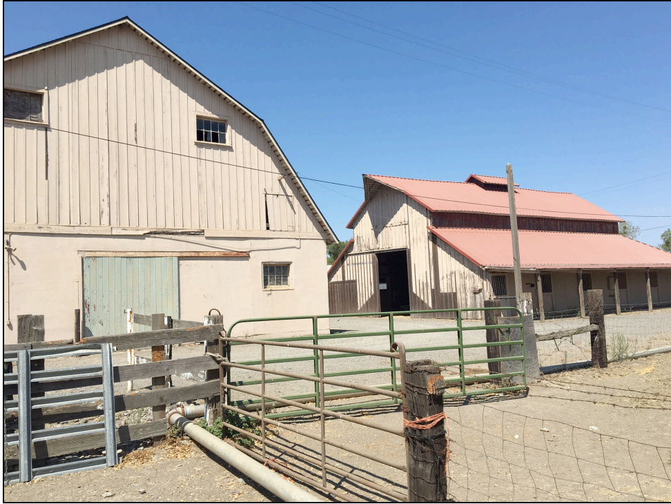
Plate 6. Barns, other out buildings, corrals, two ranch houses, and other structures occupy most of the northern part of the property. These areas are not intended for use by the public, but some parking areas are nearby.
