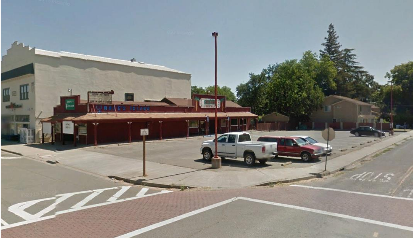
(Rose's Island Bar has been demolished, and will be replaced by the proposed project)
