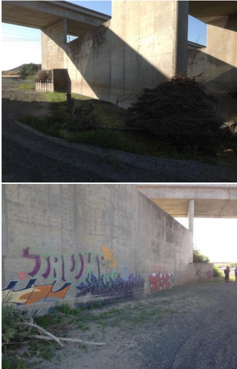
Figure 15: Photos showing I-505 Bridge piers.
