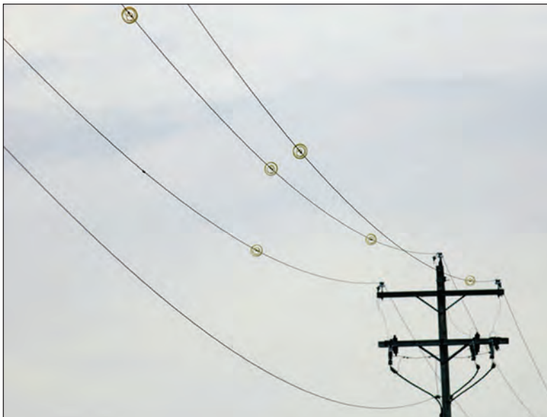
FIGURE 6.14: Swan-Flight™ Diverters installed on the phase conductors of a distribution line.
