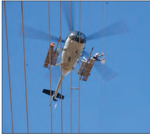
FIGURE 6.2: A helicopter crew installing line marking devices on a power line.
