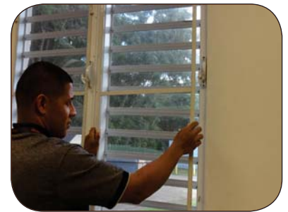
Install or repair window & door screens.
