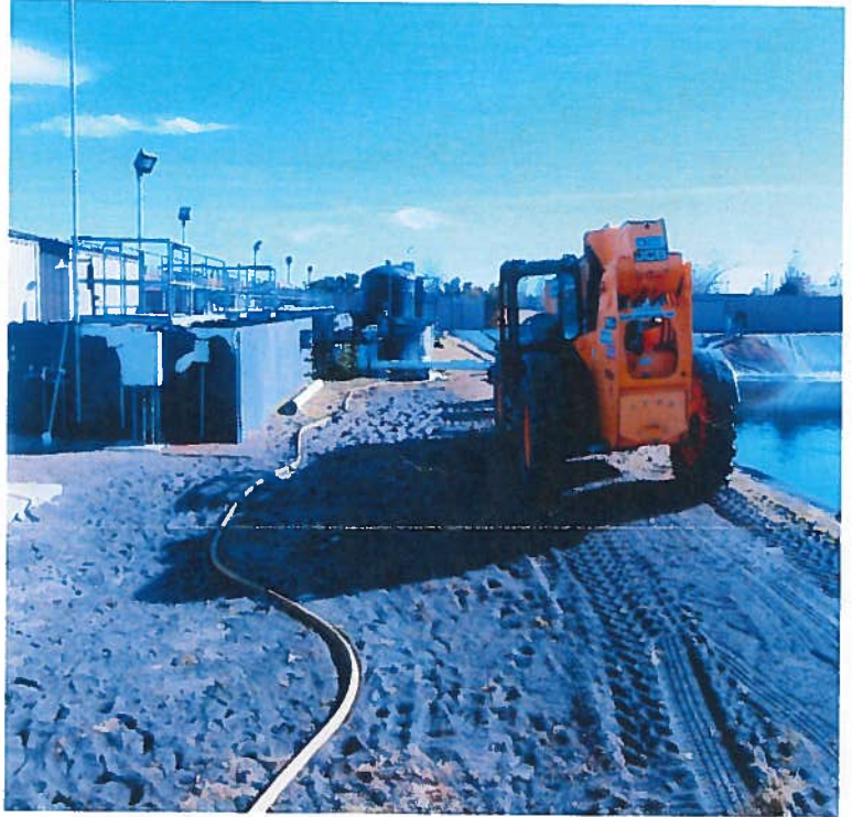
Figure 2. Tertiary filter sand dispersed to the ground between the filters (left) and the recycled water pond.
