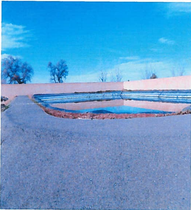
Figure 3. Emergency Storage Pond.
