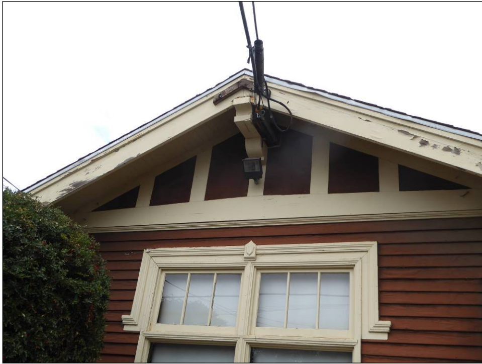
Figure 4-3 Yolo Branch Library Character-Defining Features (Gable End and Porch)
