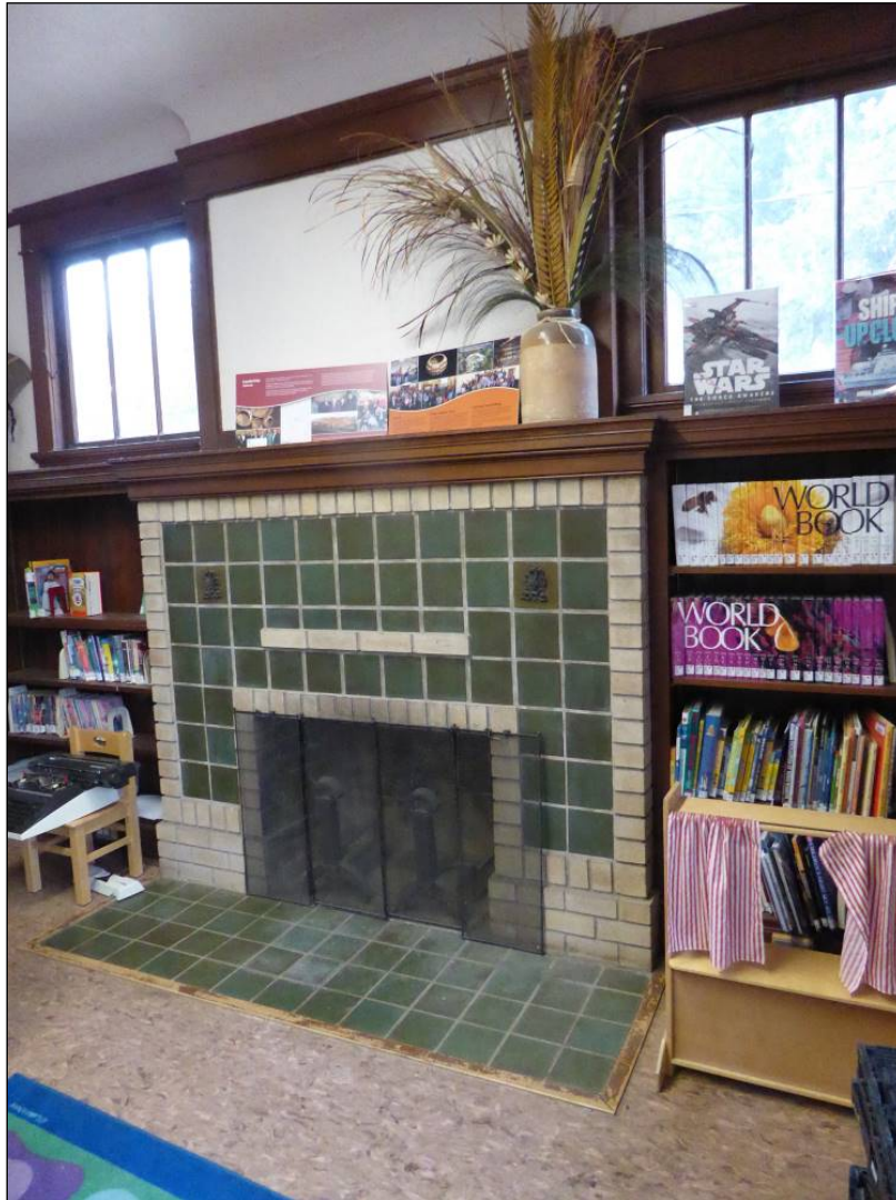
Figure 4-4. Interior eastern end fireplace with green tile and cream brick. Note the flanking bookshelves are built-in. Also partially visible is the high picture rail and cove ceiling. Image source: JRP Historical Consulting.
