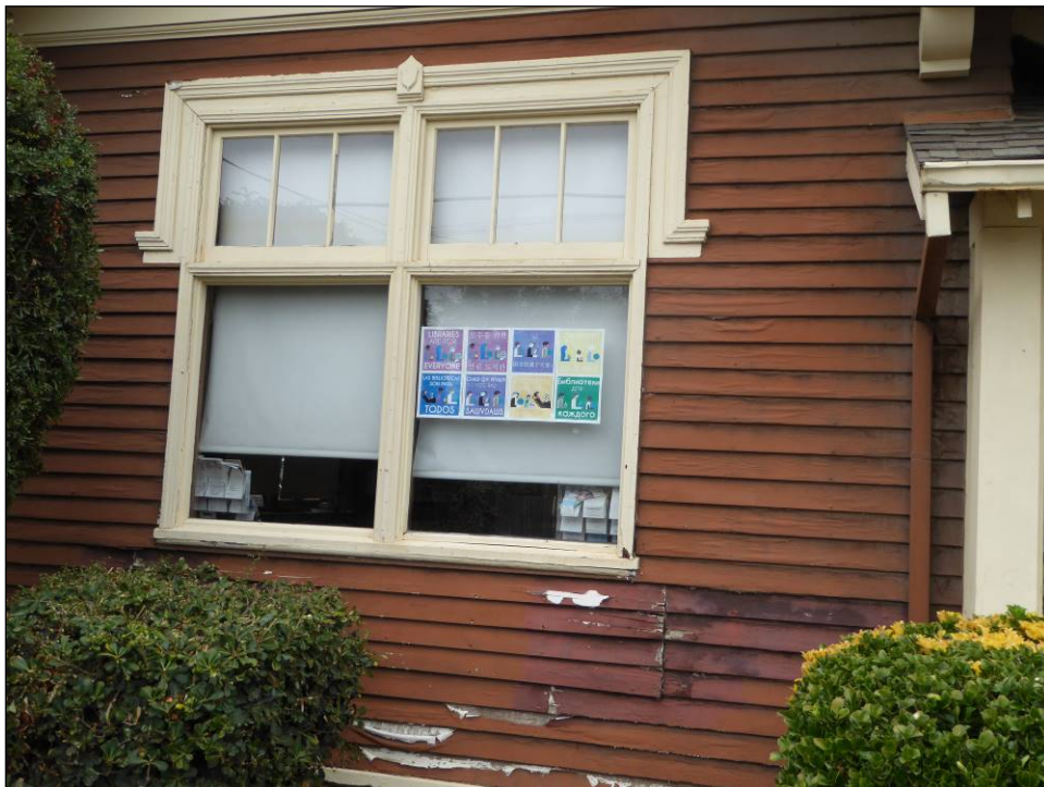
Figure 4-2. Top: Exterior of the Yolo Branch Library showing the asymmetrical cross gable plan. Bottom: Large front window with asymmetrical upper and lower sashes and square decorative hood. Image source: JRP Historical Consulting.
