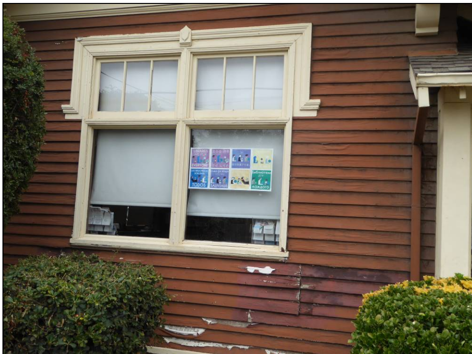
Photograph 2. Large front window, note asymmetrical upper and lower sashes with square decorative hood.
