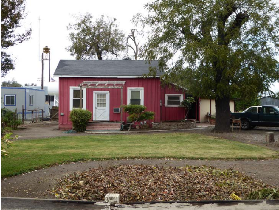
P5a. Photograph or Drawing (Photograph required for buildings, structures, and objects.)
