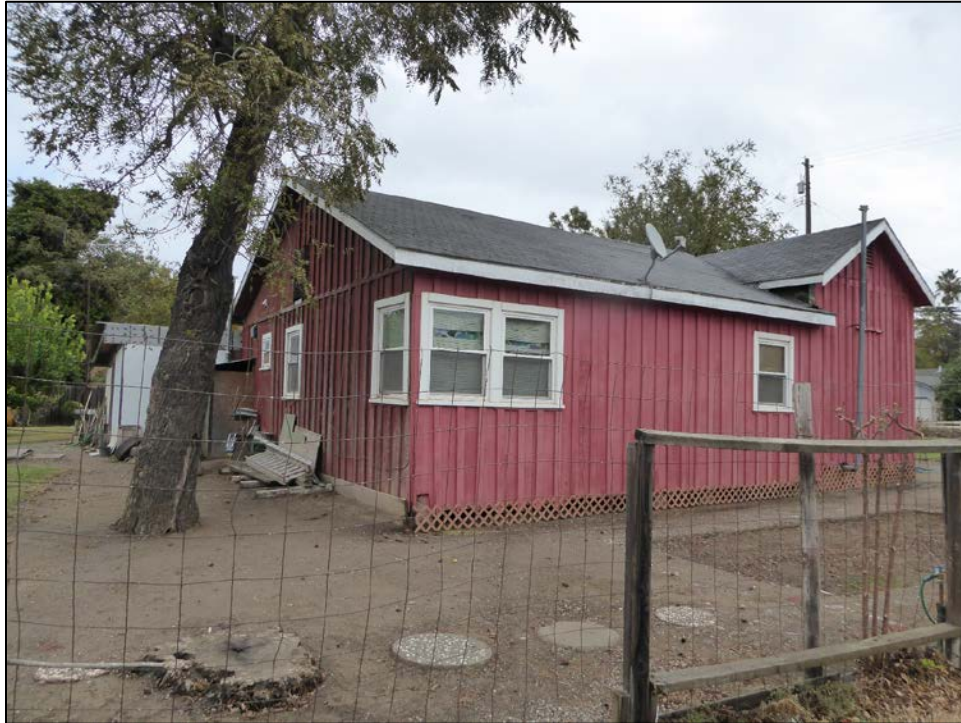
Photograph 2. Rear portion of the residence, camera facing northeast.
