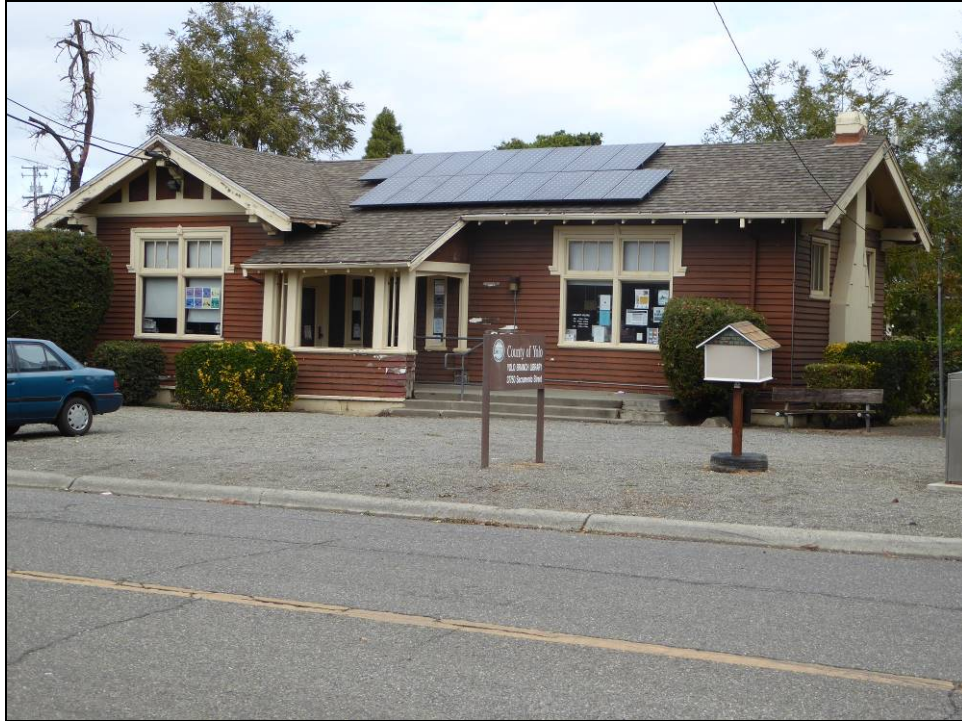
Photograph 1. Exterior of the Yolo Branch Library showing the asymmetrical cross gable plan, camera facing north.
