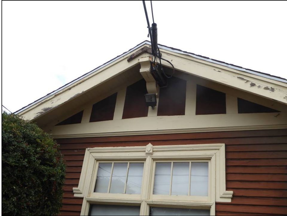
Photograph 3. Western gable end showing decorative half timbering and supporting bracket.
