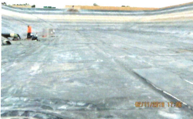
Clean liner being inspected and repaired
