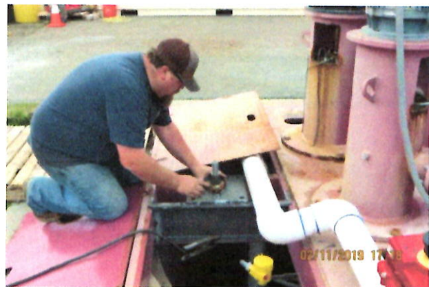
New wet well canal gate collar being assembled
