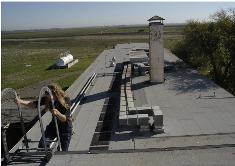
(c) On roof of East Bay looking west
