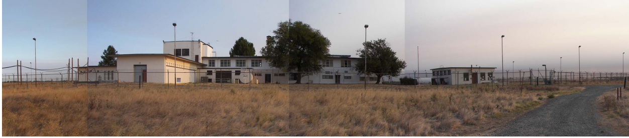
Former Davis Global Communications Site
