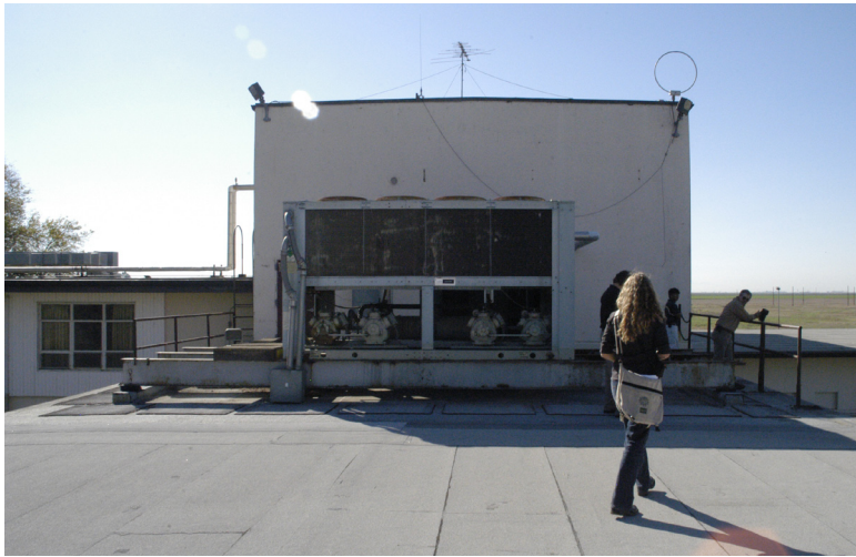
(a) On roof of North Bay looking south
