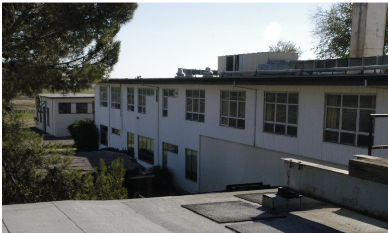
(b) On roof of North Bay looking east
