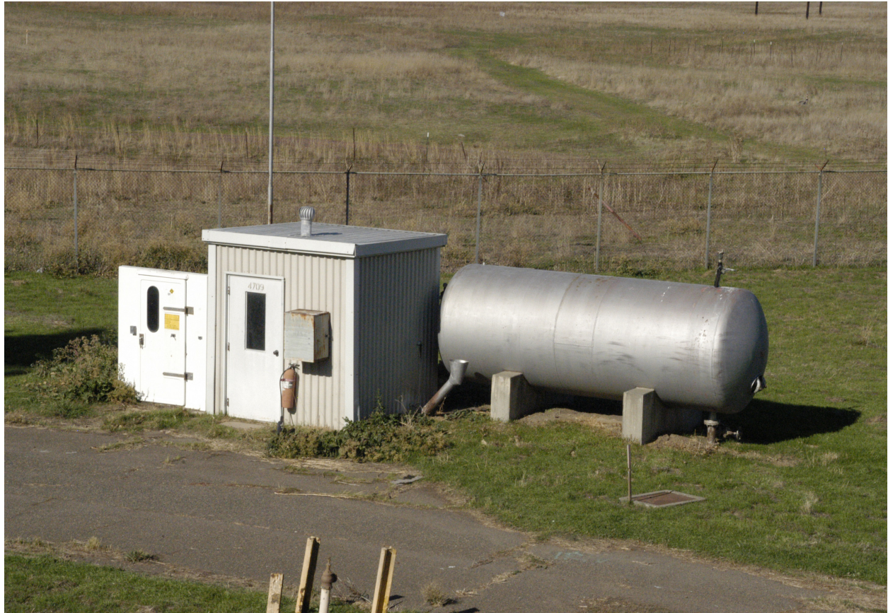
Filtration Shed, Pumphouse and Storage Shed
