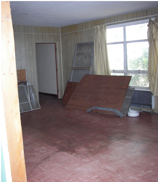
(b) Second Floor Room Typical
