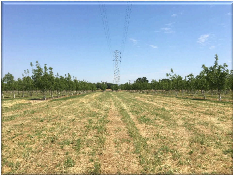
Plate 5. Looking north along the transmission line right-of-way through the center of the project site. This area will remain open following installation of the arrays.
