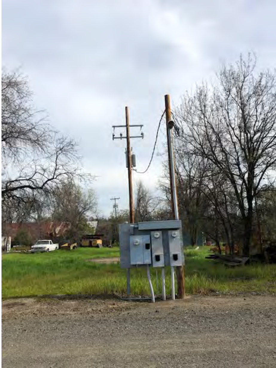
Proposed tie-in point to existing power line. View looking north.
