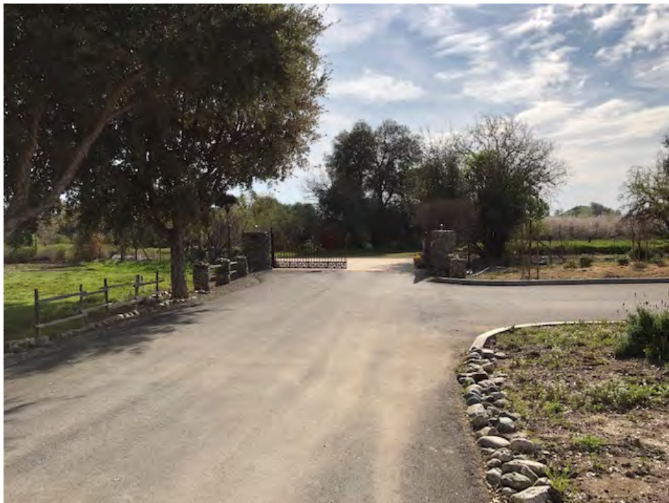
Existing paved access road to proposed tower project site and tie-in point to existing underground fiber-optic communications line. View looking east.
