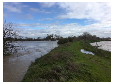
Flooding in Yolo County
