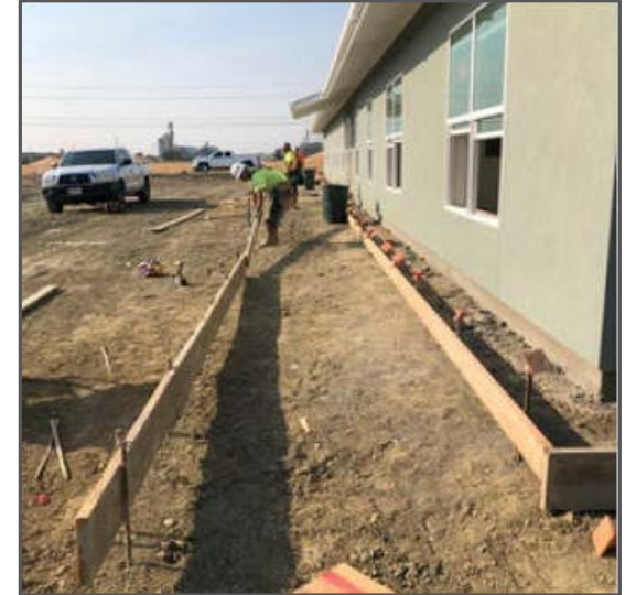
102/Beamer Emergency Shelter Construction
